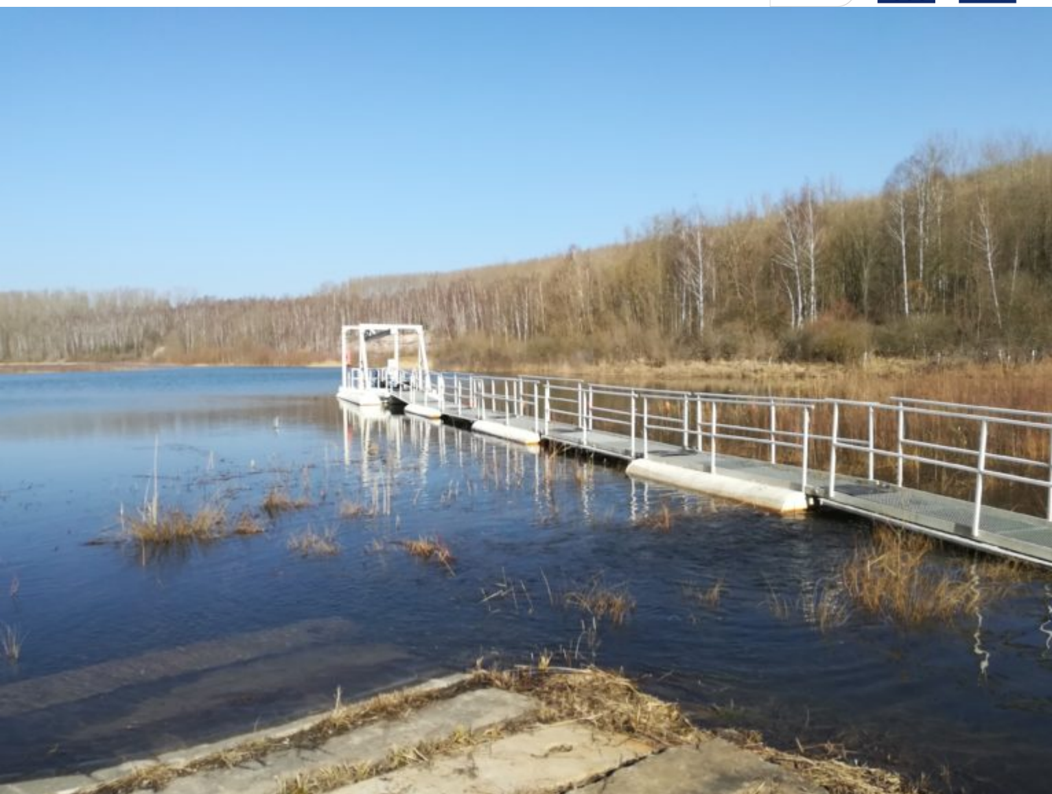
Pumpstation am Restloch Zechau III
