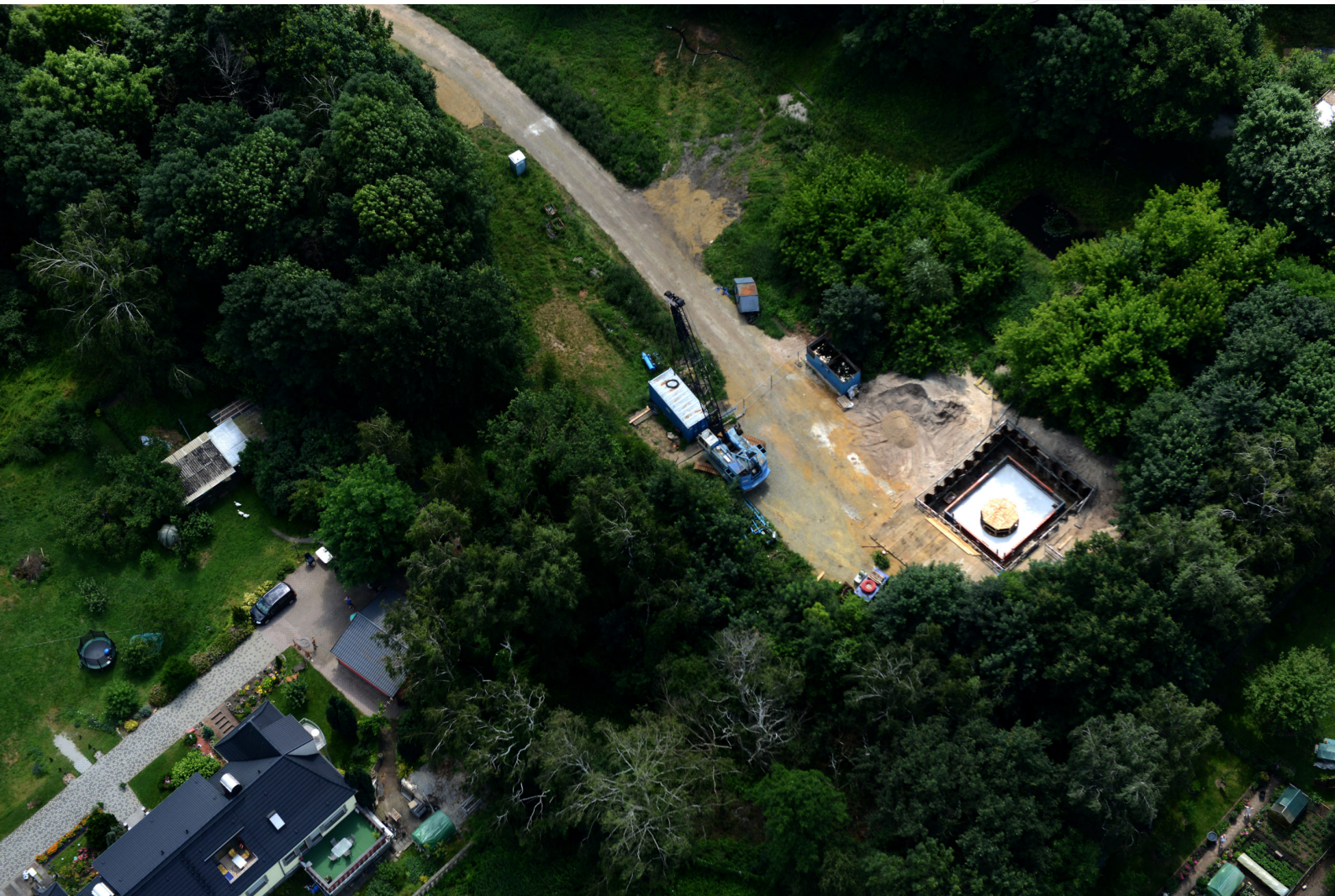
Baugrube des HBr 4 in Senftenberg | P. Radke | 2013
