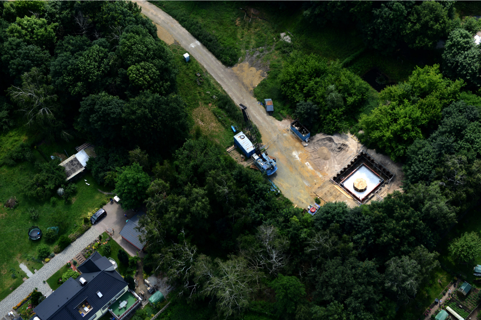
Baugrube des HBr 4 in Senftenberg | P. Radke | 2013
