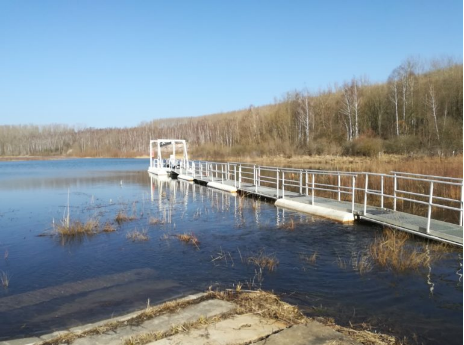
Pumpstation am Restloch Zechau III
