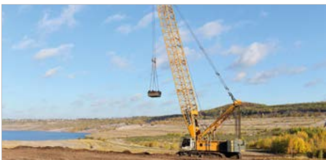
Drop-plate compaction in the former mining area of Wulfersdorf
