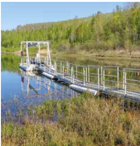
Pumpstation am Restloch Zechau III
