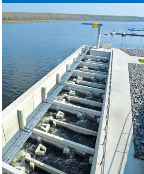
Fish ladder at river Mulde reservoir
